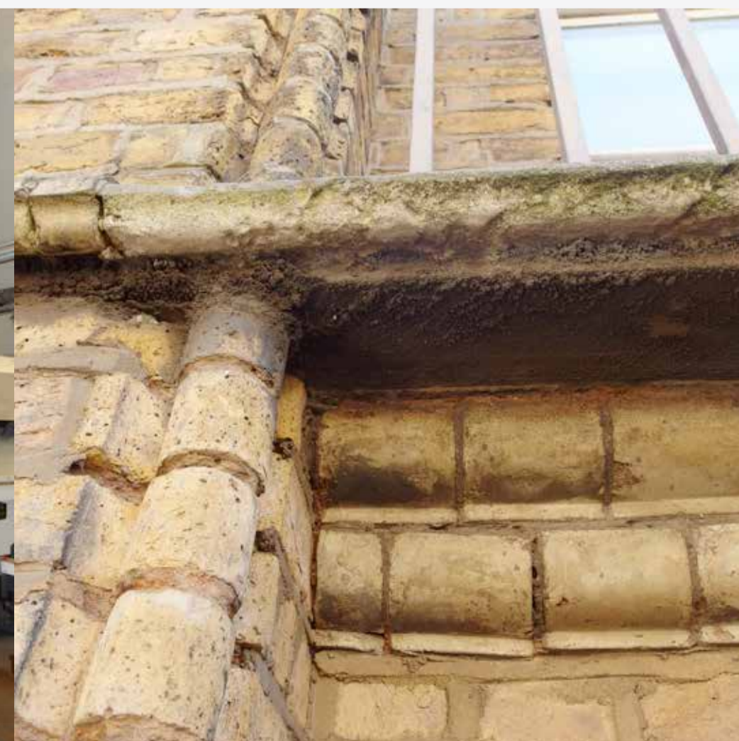
Crumbling sills and other features to be repaired.
