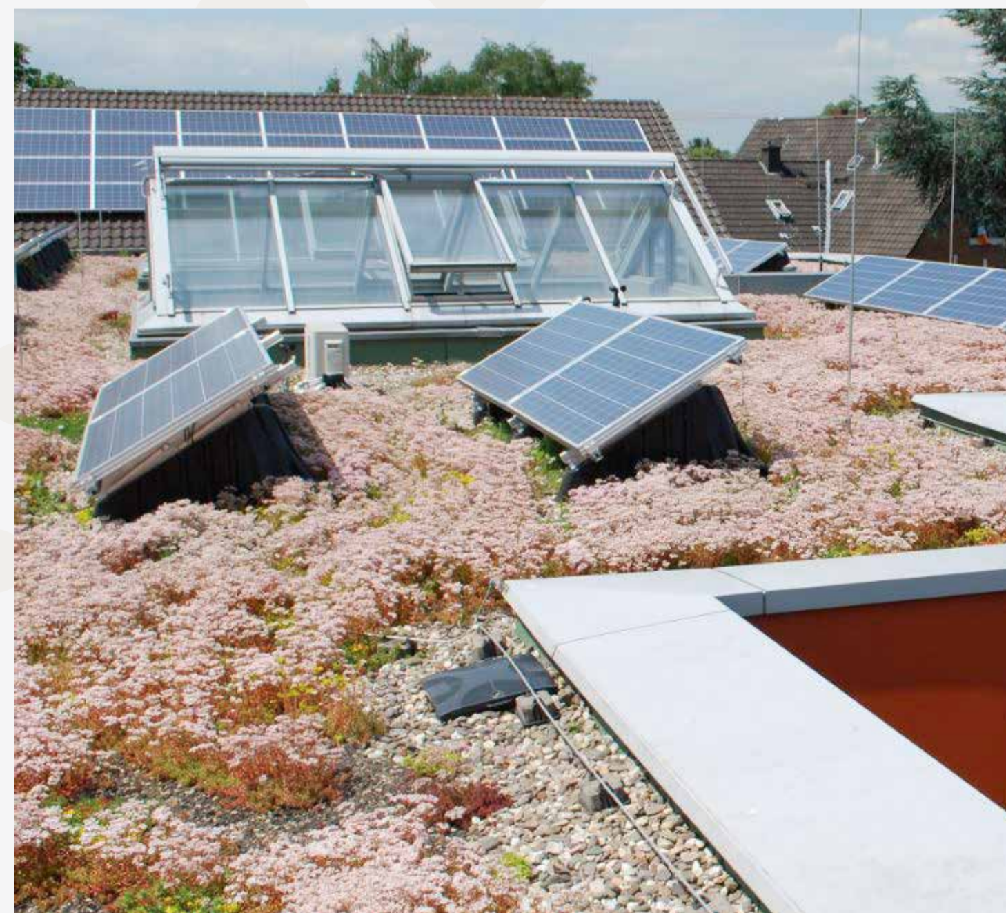
Green roofs with photo-voltaic panels.
