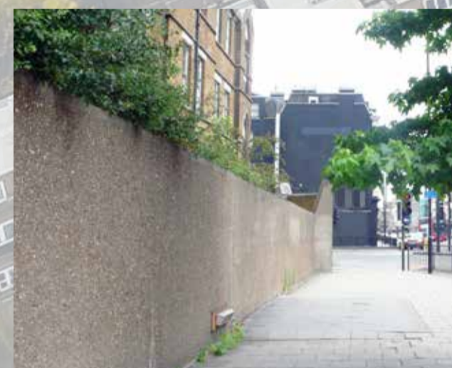
The concrete wall creates a barrier to the site.
