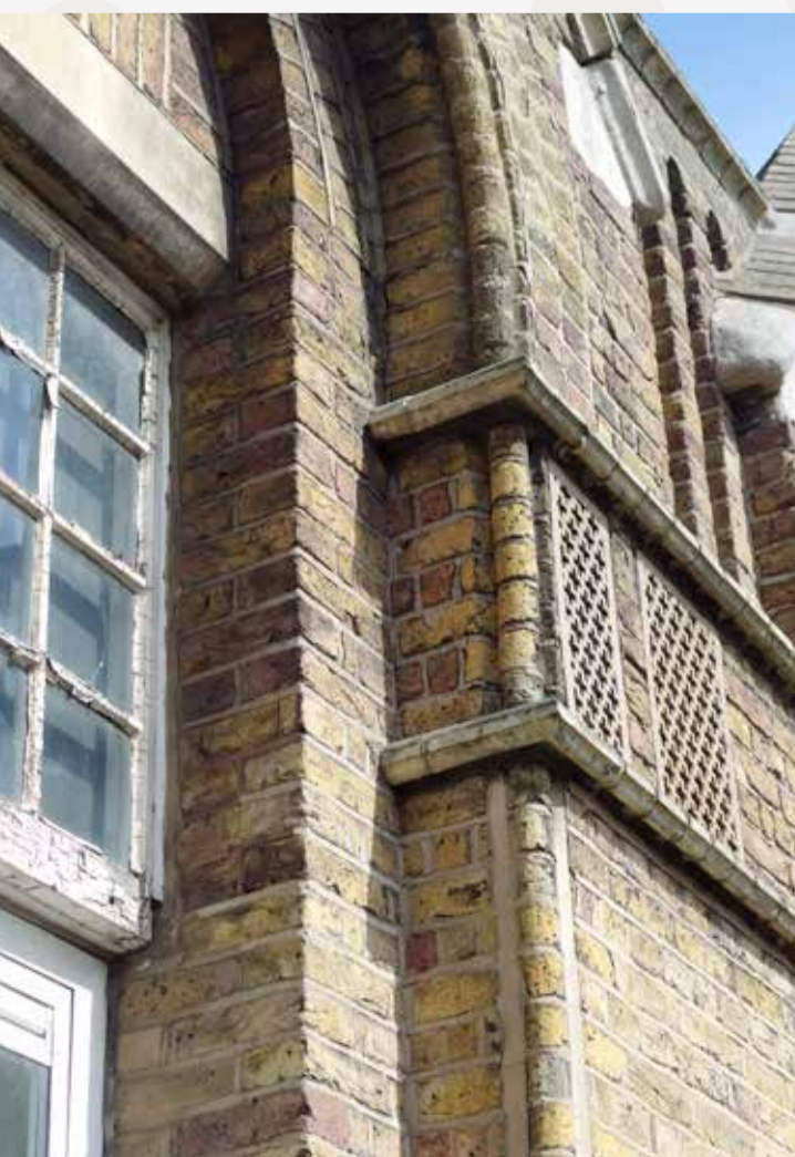
Windows and pointing to be replaced.
