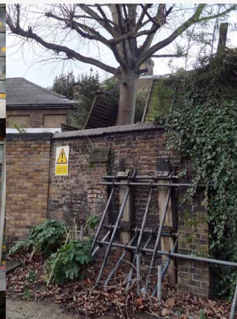
Retaining walls to be repaired.
