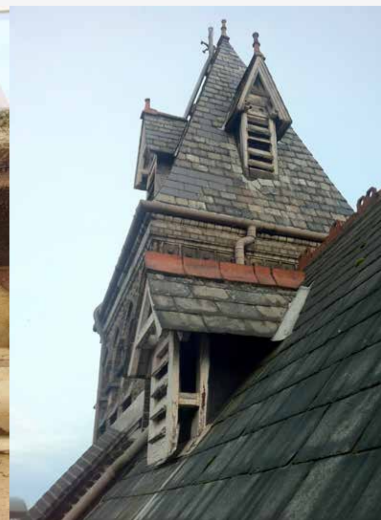
Woodwork to be cleaned and repainted.
