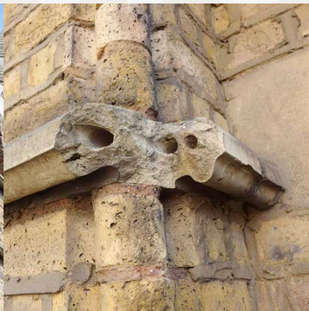
Damaged brickwork to be repaired.
