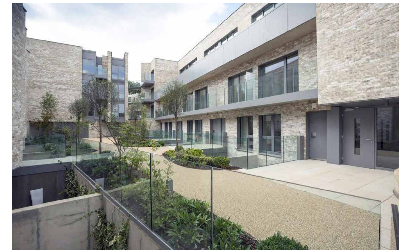
Attractive residential courtyard with well placed planting.
