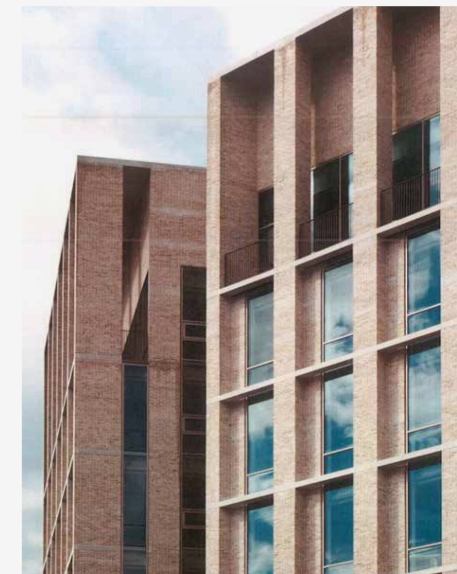
High-quality brickwork and well proportioned façade.
